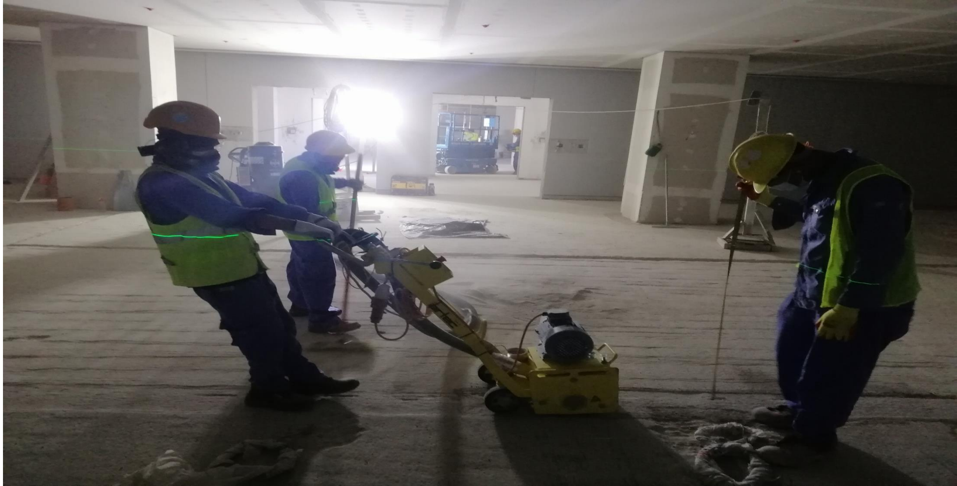
Scarifying Machine Cutting to achieve required FFL.
